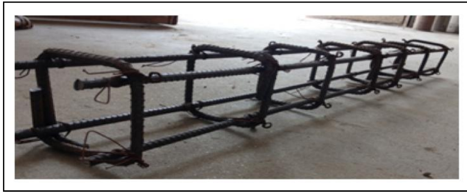
Fig.6 Reinforcement of beam
